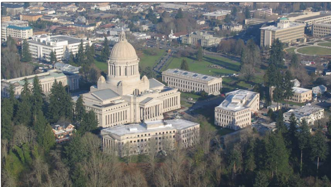
Looking NE - December 2005
