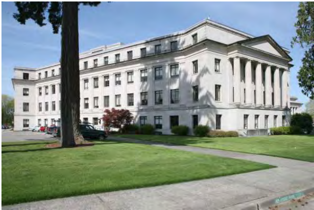
Southeast and east facades
