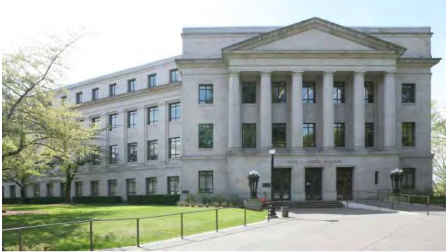
North portico and partial NE facade
