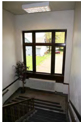
Stairwell, looking east
