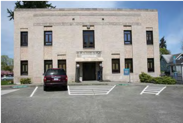
South (rear) facade
