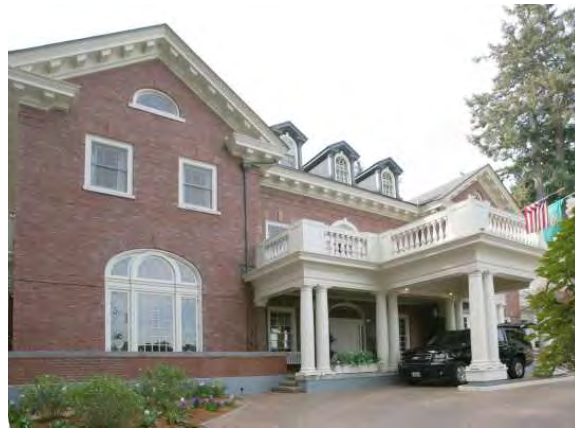
Front (north) facade
