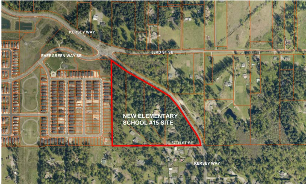
Figure 1.1 – Elementary School No.15 Neighborhood Aerial - 57 th St. SE / Kersey Way, Auburn WA
