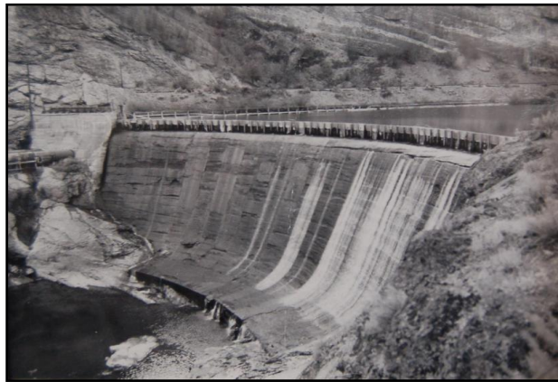
Figure 7. Dam Falls with unknown low (leakage) flow from 1950s (from Similkameen River Trail Facebook Page).
