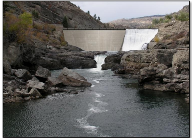
Figure 18. Simulated photo of 120 cfs over one-third of Dam Falls and over Similkameen Falls.
