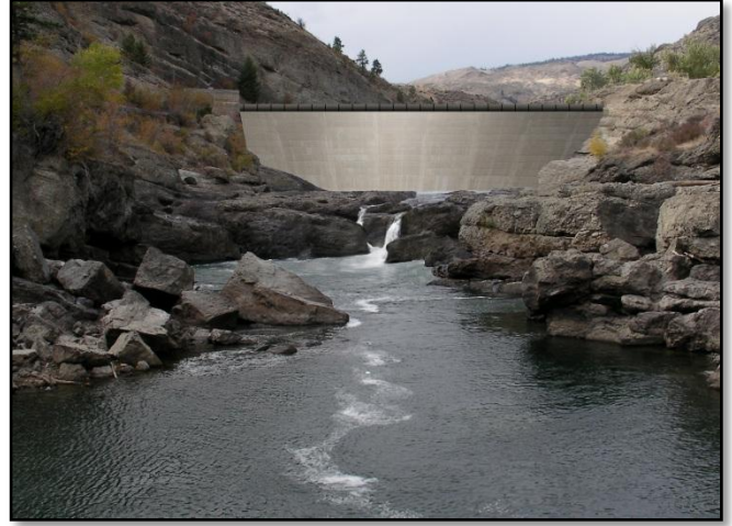
Figure 16. Simulated photo of 0 cfs over Dam Falls and 30 cfs over Similkameen Falls.
