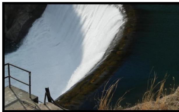
Figure 21. The Dam Falls at 700 cfs showing nappe separation (where falling water becomes aerated).
