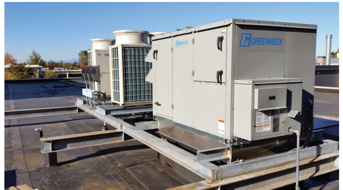
Mechanical Upgrades & Replacements, South Seattle College
