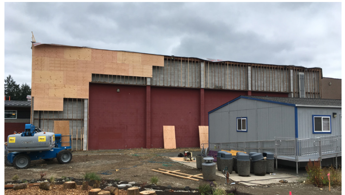
Envelope Improvements, Capital High School, Olympia School District
