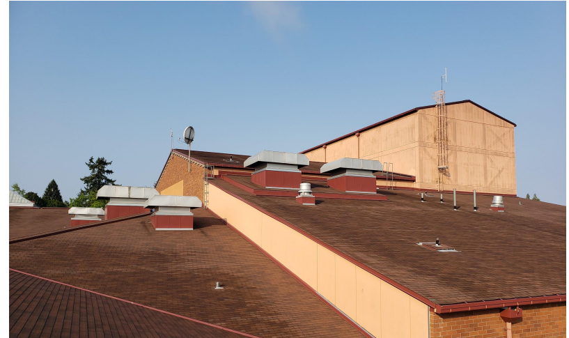
MTH roof hoods & mech stanchions (2012)
