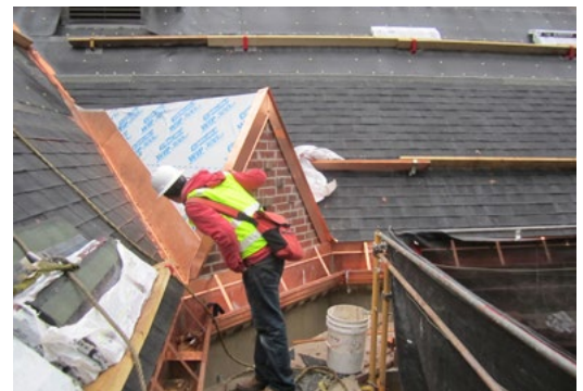
University of Washington, Lewis Hall roof improvements
