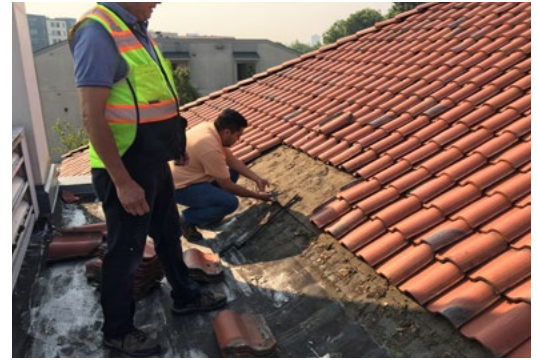
Green Lake Branch Library roof repairs
