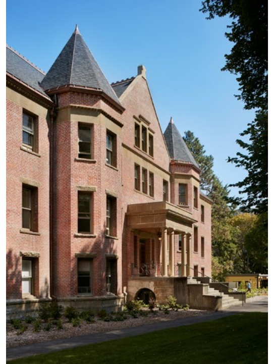
Roof replacement and masonry restoration of UW Lewis Hall.
