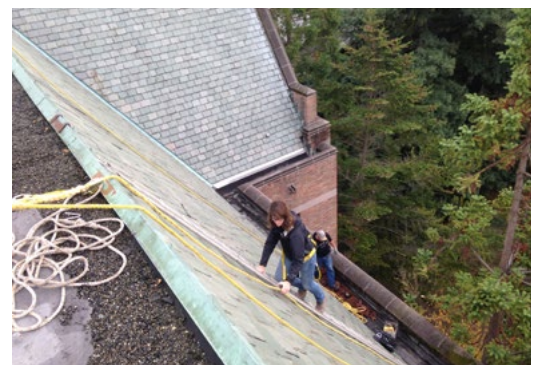
Slate roof repairs at Anderson Hall, University of Washington
