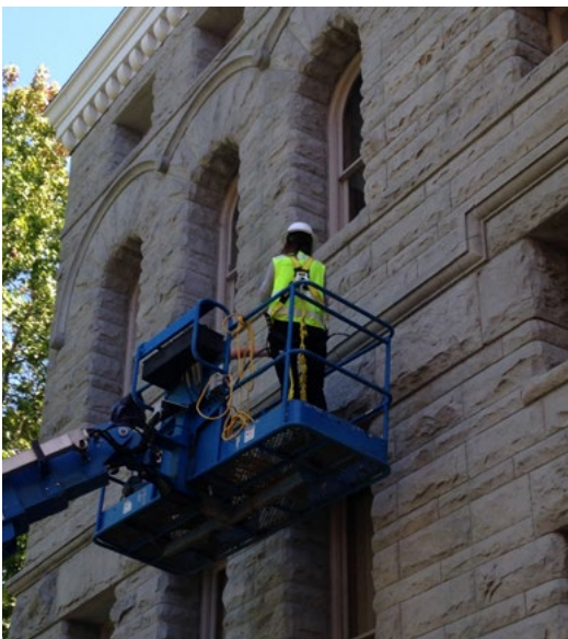
Pia Westen performing masonry investigation at Old Capitol Building.
