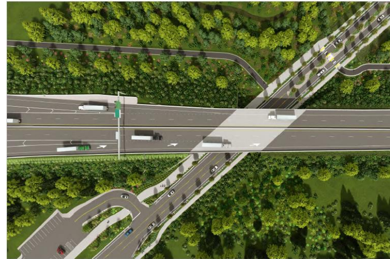
SR 167 Expressway Bridge over 20th St. E.
