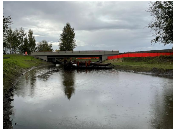
New Fish Passable bridge over Hylebos Creek (Stage 1b)
