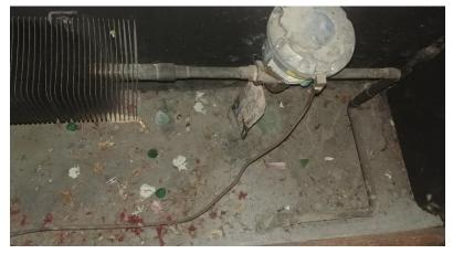
Radiator and Pneumatic Control Valve. Shows HW piping buried in concrete
