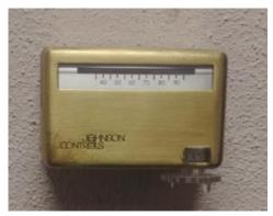
Pneumatic Thermostat (Installed in 1987)
