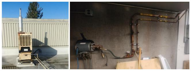
Diesel Generator on Roof and fill piping in lower mechanical room
