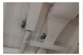
VAV Boxes (box with a pneumatic damper)
