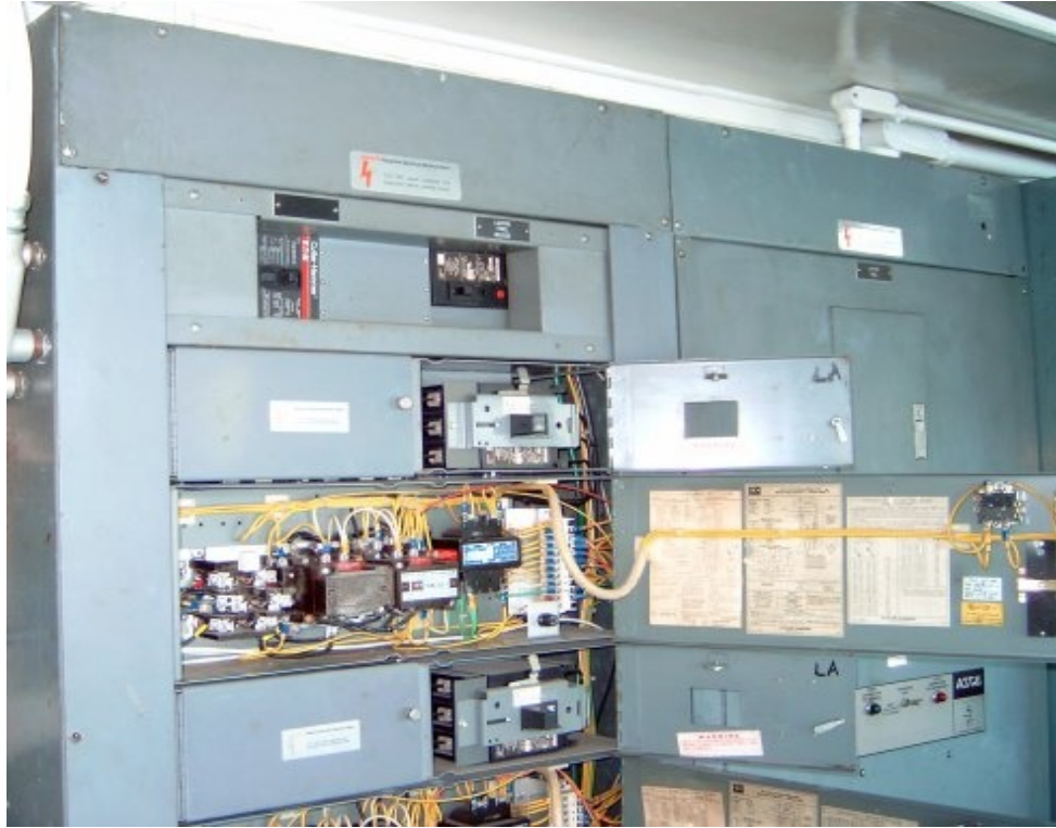
Figure 8 Power Distribution Section (Right) Motor Control Center – with compartments opened (Left)
