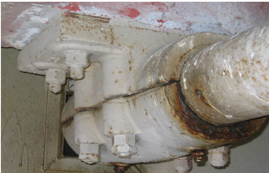
Figure 2 West Gate Pillow Block Bearing
