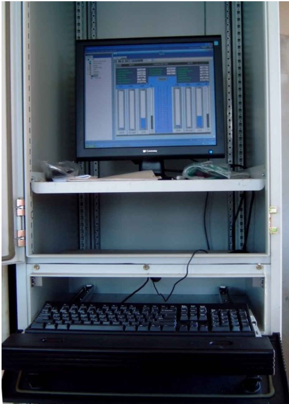
Figure 5 METASYS Operator Station (MMI)
