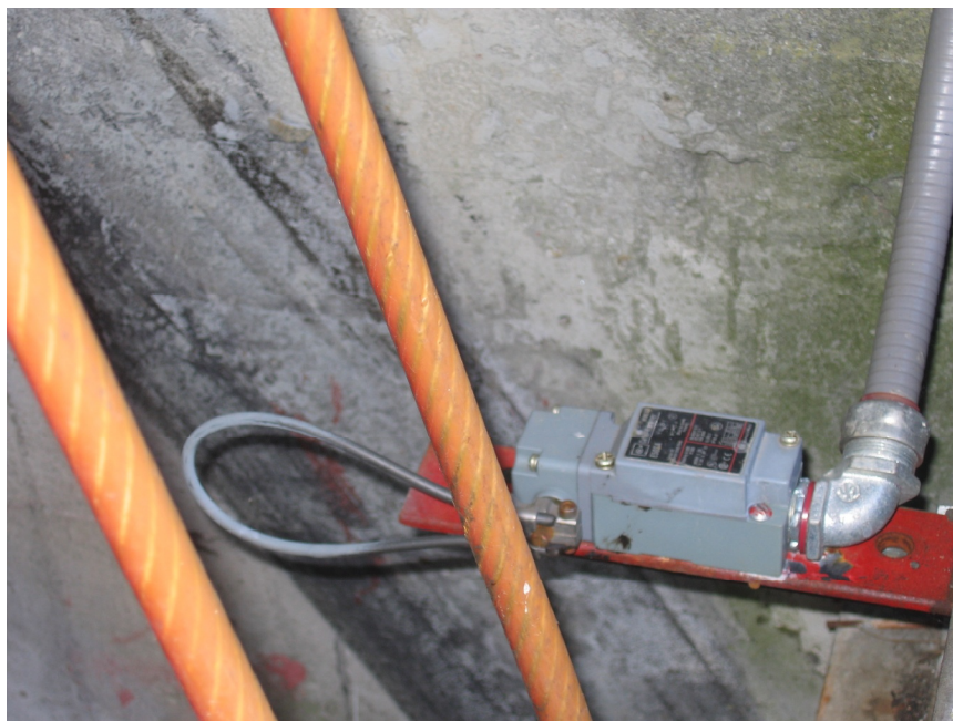
Figure 7 West Gate Back-Up Limit Switch
