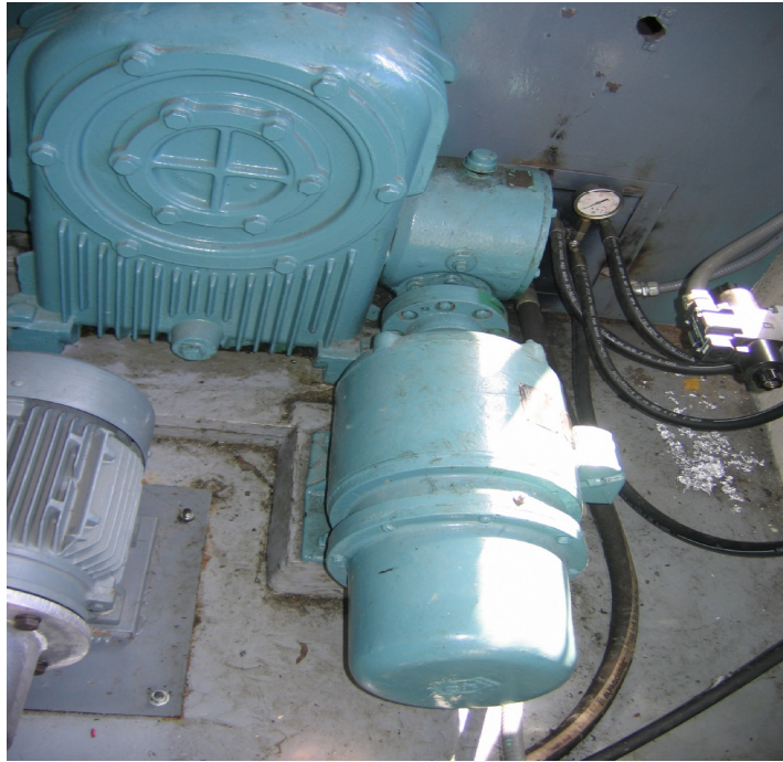
Figure 3 West Gate Motor & Reducer
