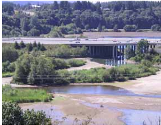
South Basin and I-5 Bridge during Drawdown
