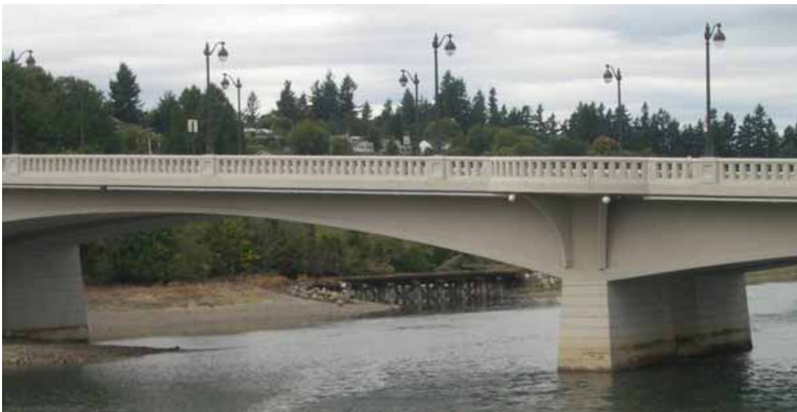
Figure 3: Recently Constructed Fourth Avenue Bridge
