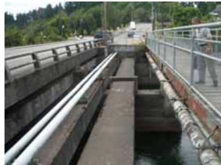
Utility Lines at Dam
