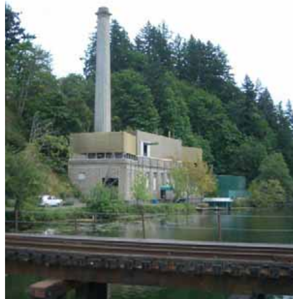
General Administration Powerhouse
