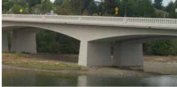
4th Avenue Bridge Pier to be Extended Down
