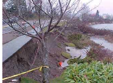
Deschutes Parkway slope failure after the Nisqually Earthquake
