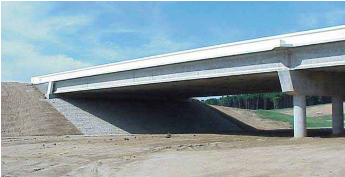
Figure 2: Precast Concrete Girder Bridge
