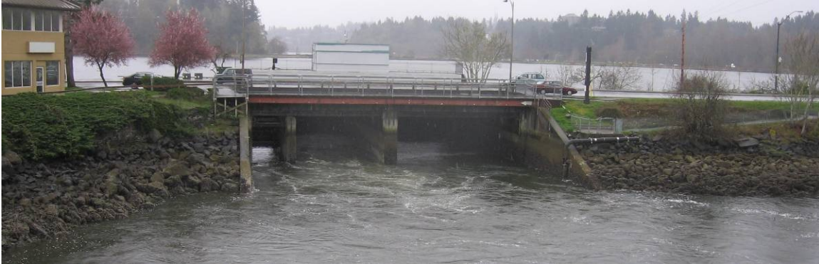
Figure 10. Capitol Lake Dam
