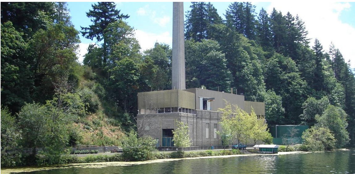
Figure 11. General Administration Powerhouse
