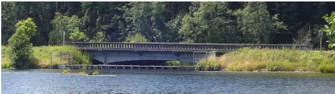
Figure 9. Percival Cove Bridge
