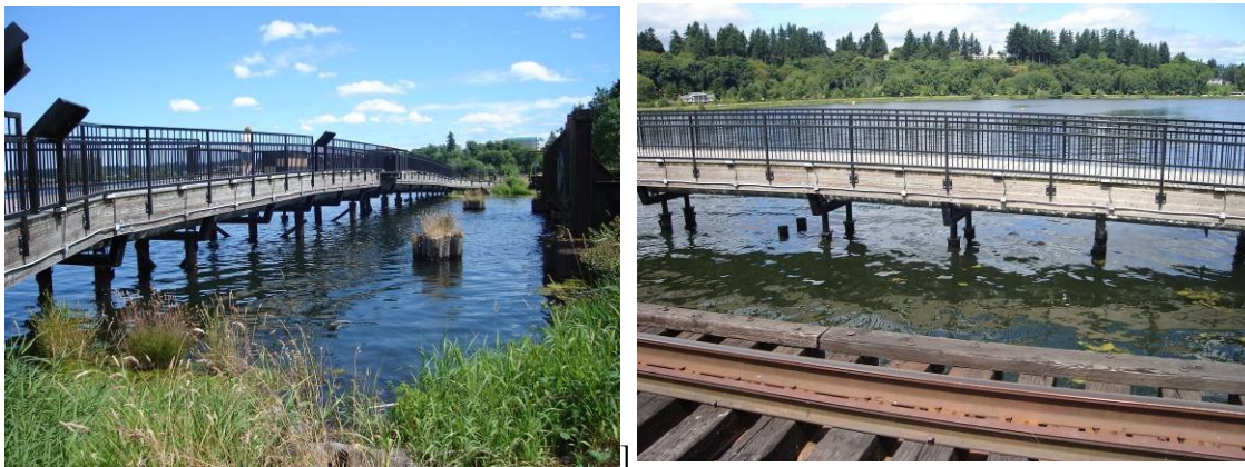
Figure 8. Pedestrian Bridge, located next to BNSF Railroad Trestle
