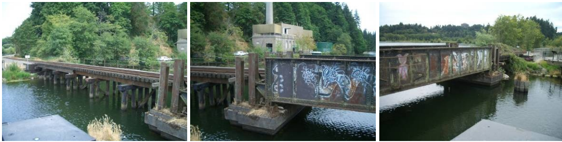
Figure 7. BNSF Railroad Trestle
