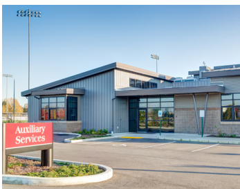
Auxiliary Service Building Whatcom Community College Bellingham, WA
