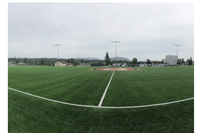
Soccer Field Renovation Skagit Valley College Mount Vernon, WA
