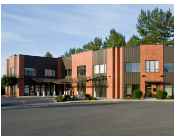
Foundation Building Whatcom Community College Bellingham, WA
