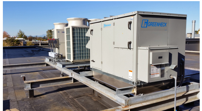
Mechanical Upgrades & Replacements, South Seattle College
