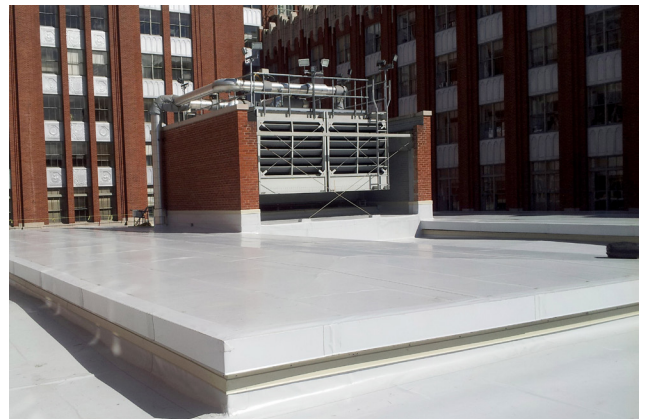
US GSA FEDERAL OFFICE BUILDING NEW ROOF
