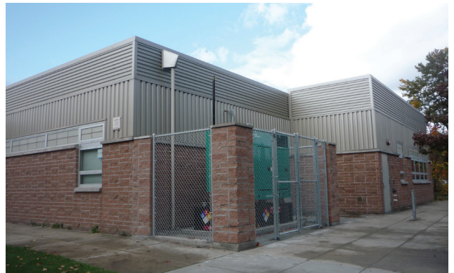
EDMONDS SCHOOL DISTRICT | MEADOWDALE HS GENERATOR
