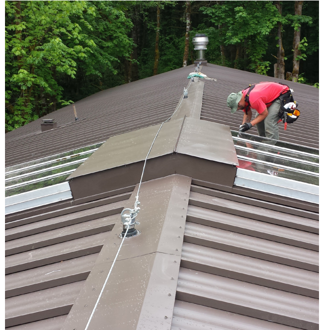
THE EVERGREEN STATE COLLEGE | ROOF ASSESSMENT
