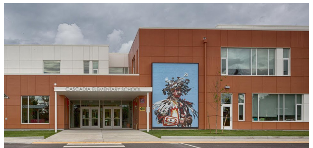
SEATTLE PUBLIC SCHOOLS CASCADIA ELEMENTARY SCHOOL CONDITION ASSESSMENTS
