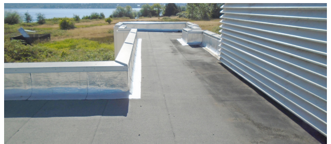
NOAA WRC | ROOF ASSESSMENT
