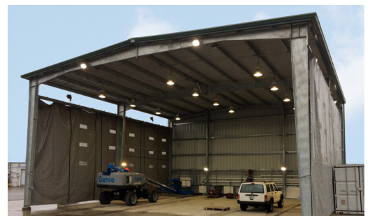
KCSW CAT SHACK REPLACEMENT
