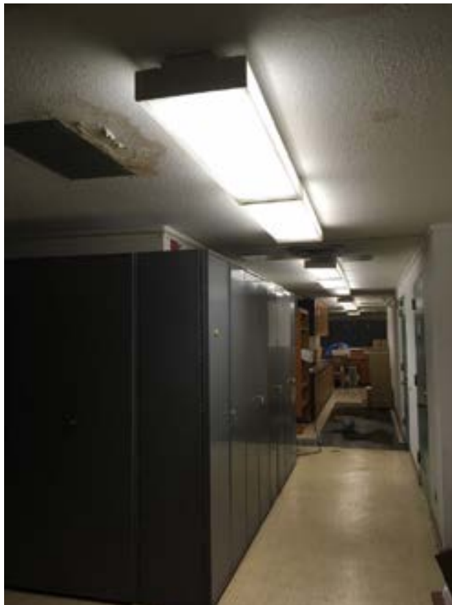
Building 10 – Service Corridor
