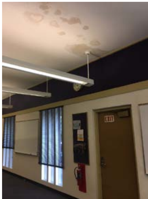
Building 10 – Classroom Leak
