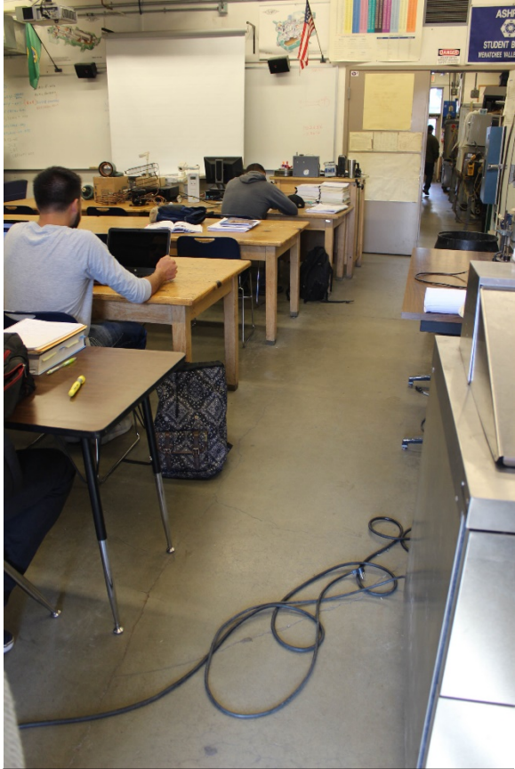
Cords across the floors cause trip hazards
