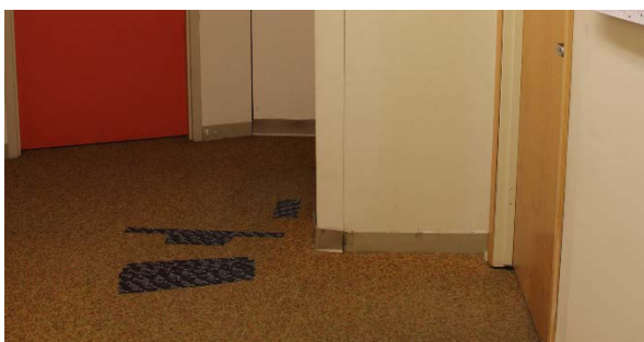
Flooring is taped up
