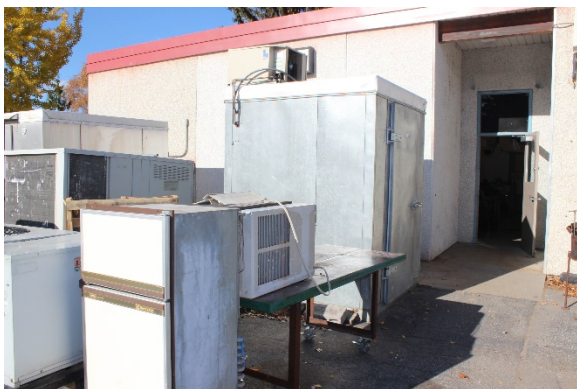
HVAC units are stored outside of building due to lack of storage space inside
