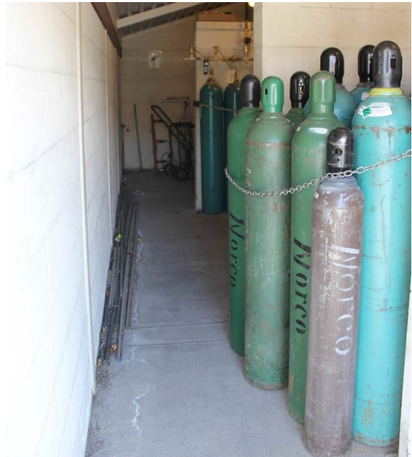
Gases are stored on the side of the building
