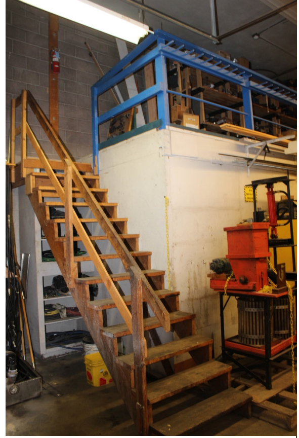
Storage closet is extremely cramped with low ceilings and minimal storage
