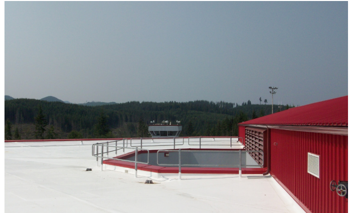
Clallam Bay Corrections Center Roof Replacement
