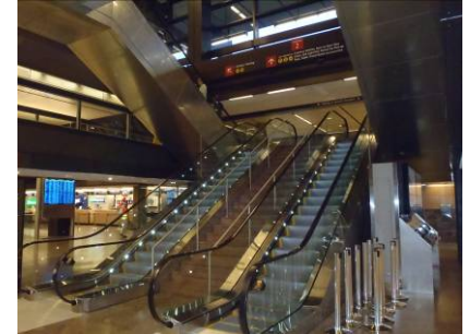
Sea-Tac International Airport Escalator Replacement and Modernization, SeaTac, WA
