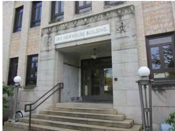
Detail of north entry
