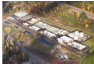
King County Brightwater Treatment Plant GC / CM
