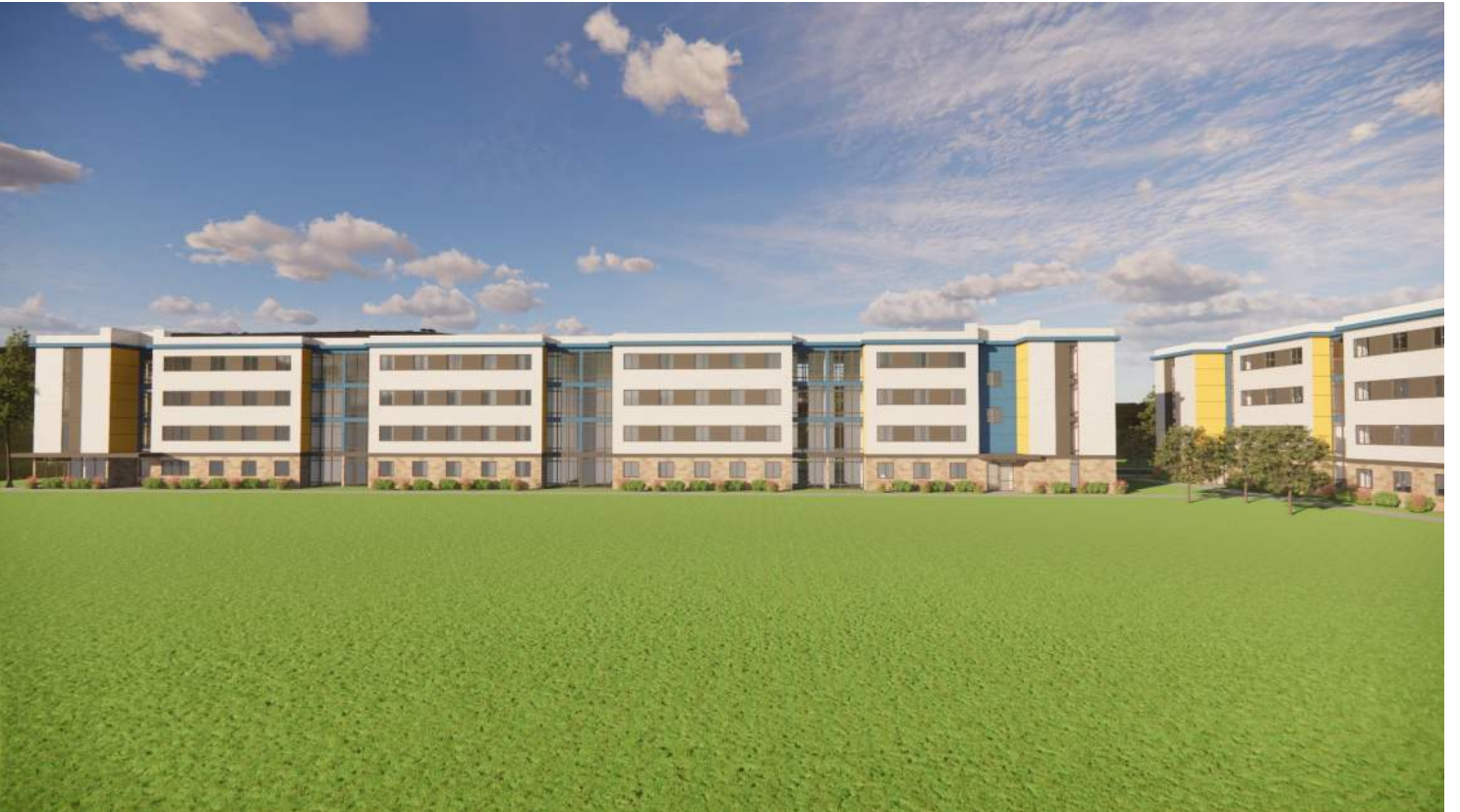
VIEW LOOKING NORTH
