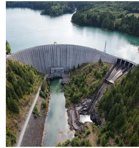
Alder Unit 11 Rebuild
