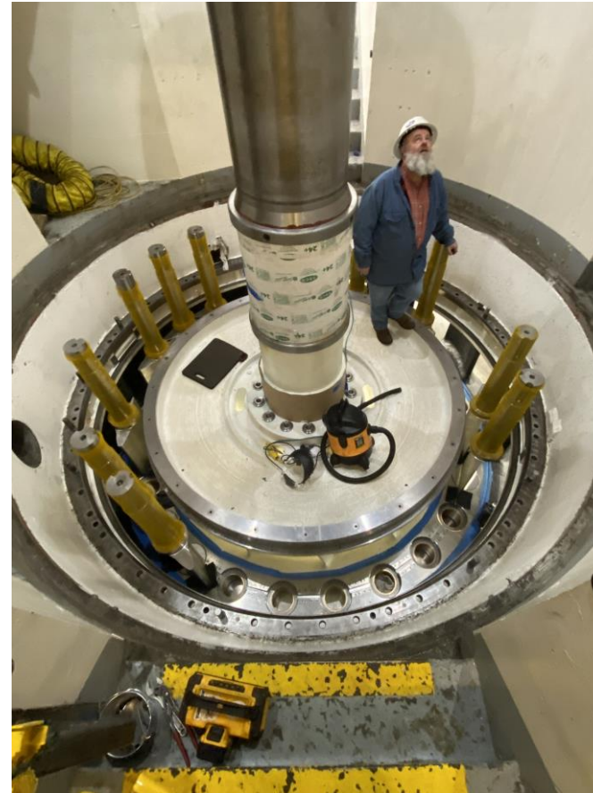
• Turbine wicket gates being installed
