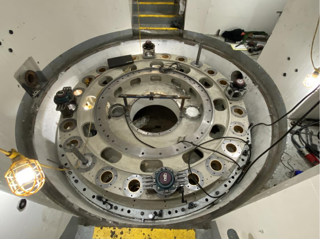
• Turbine Head Cover installed
