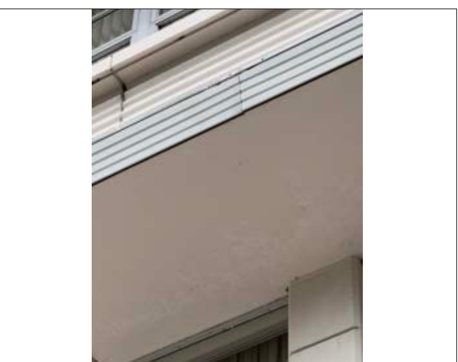
Frieze, aluminum showing a detail of the upper south facade canopies.
