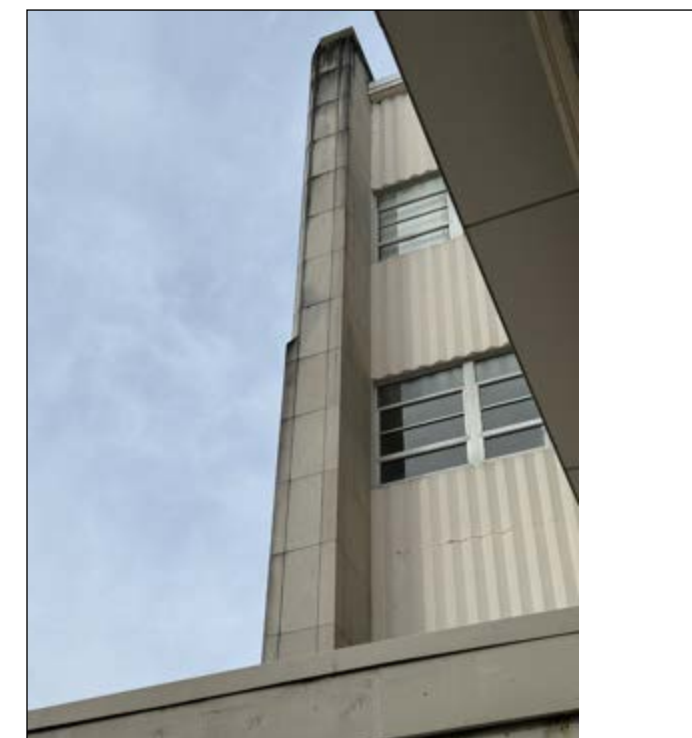
Panels, Wilkeson sandstone at the south end of the facade.
