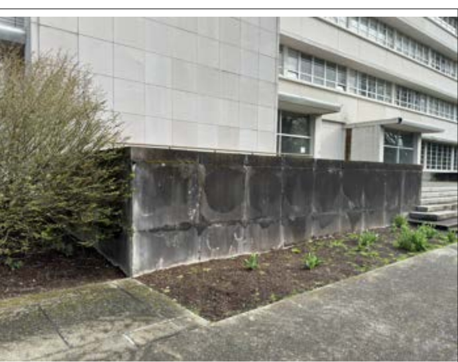
Panels, Wilkeson sandstone, showing both the railing and wall panels.
