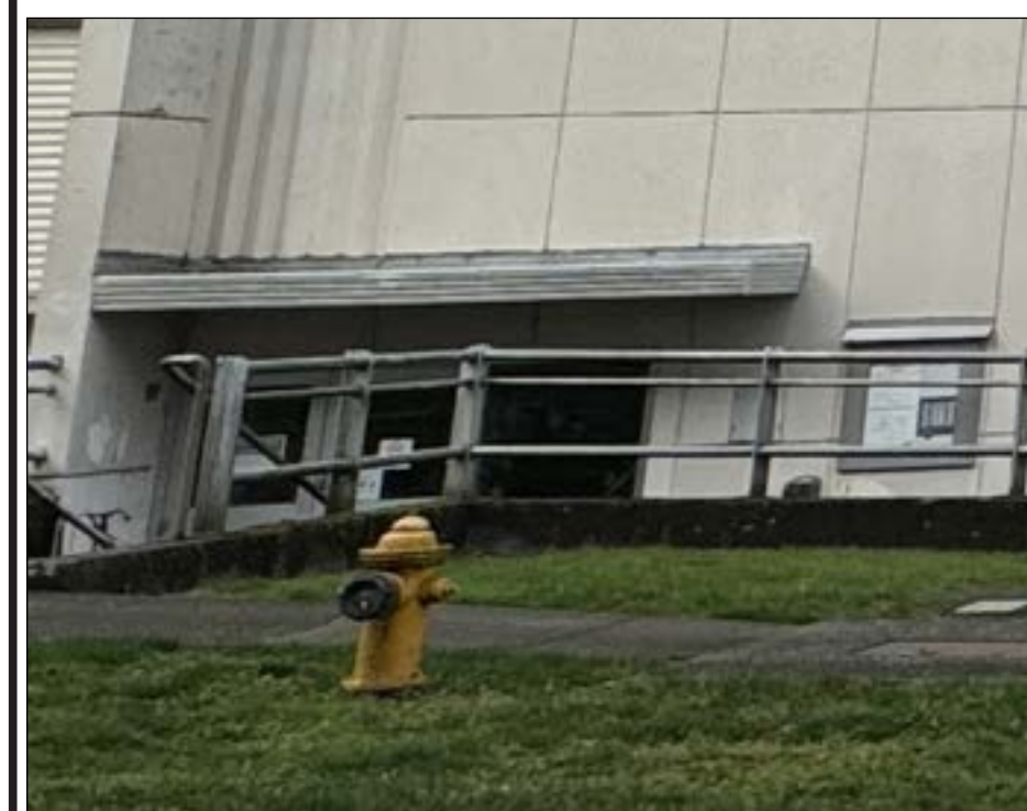
Frieze, aluminum at the entrance canopies and the railing, aluminum.
