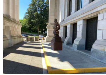
Location 3 South portico Exterior existing slab
