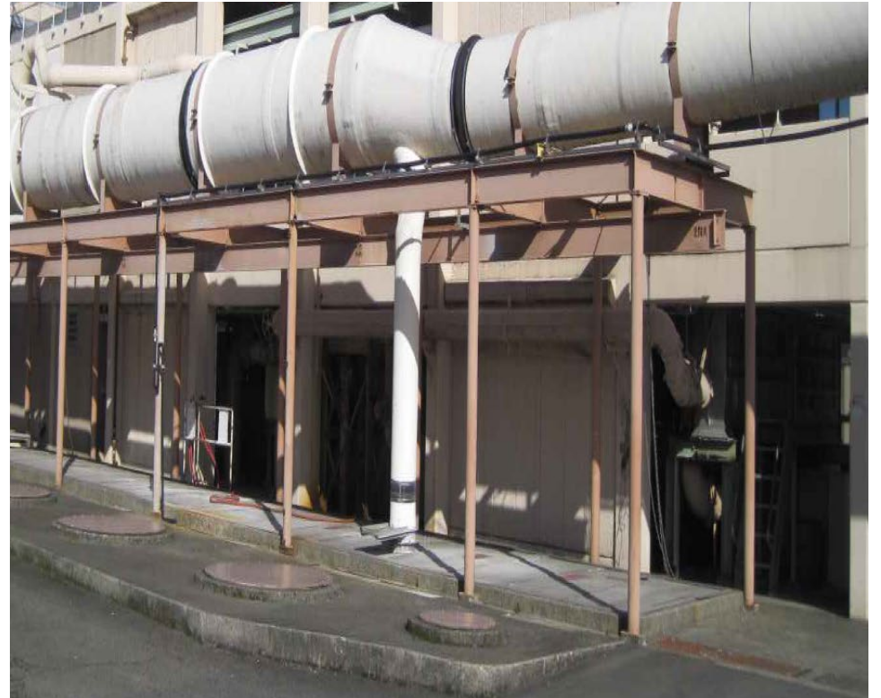
Aboveground view of the Division Channel
