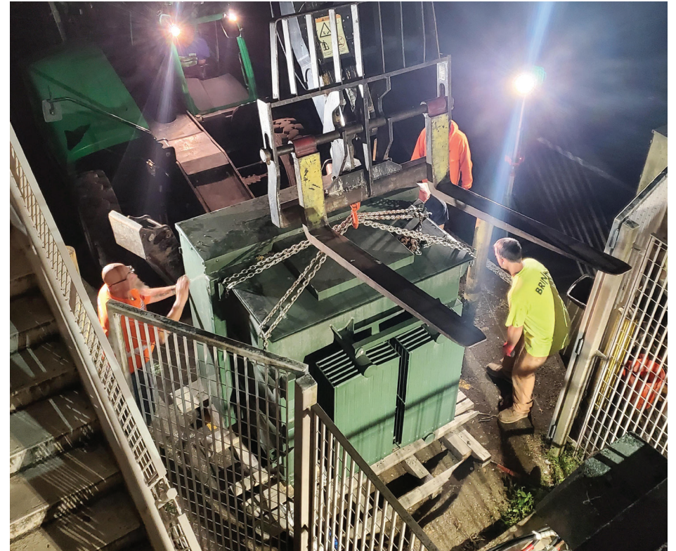
Off-hours installation of the 2900 Building Transformer
