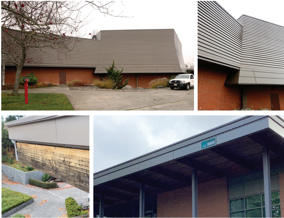
Top: Completed mansard roof with new metal panels; Bottom Left: Weathered glulam beam prior to repairs; Bottom Right: Glulam beam wrapped in low-maintenance aluminum composite panels
