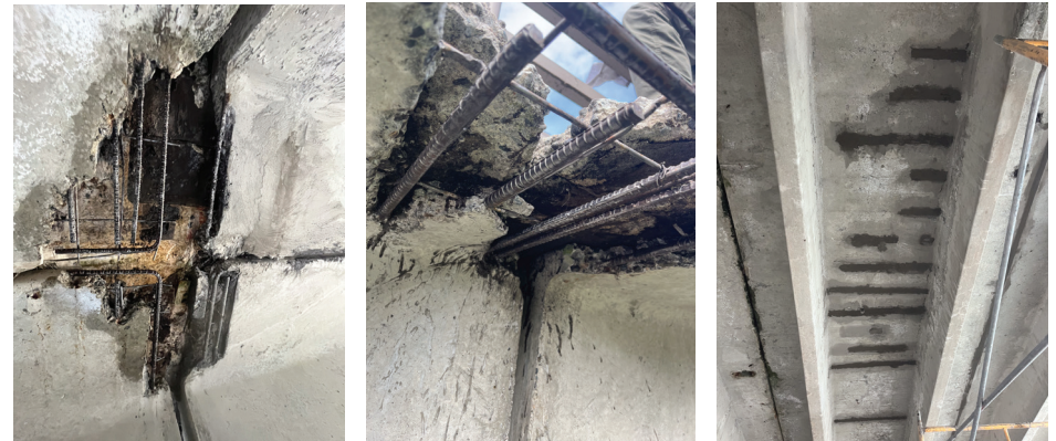
Left: Active cracking with exposed, corroded steel; Middle: Exposed reinforcing steel cleaned and prepared for repair; Right: Patch repairs along the underside of the concrete deck
