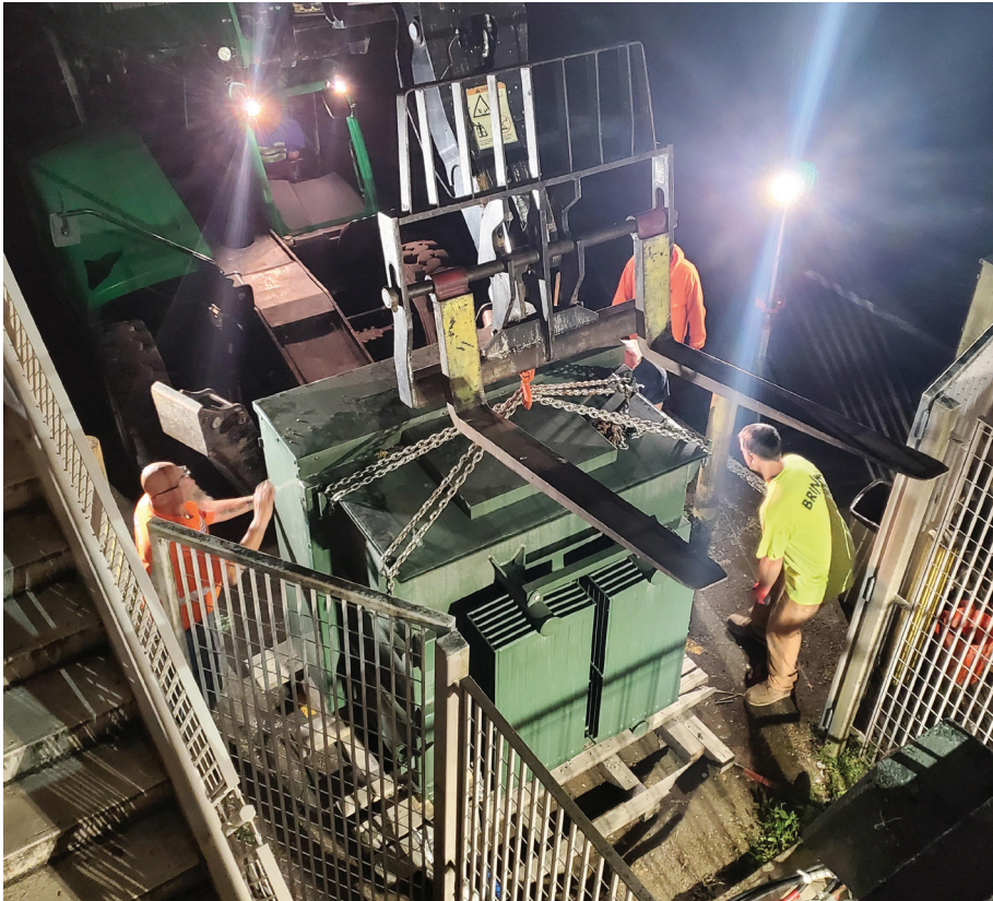
Off-hours installation of the 2900 Building Transformer
