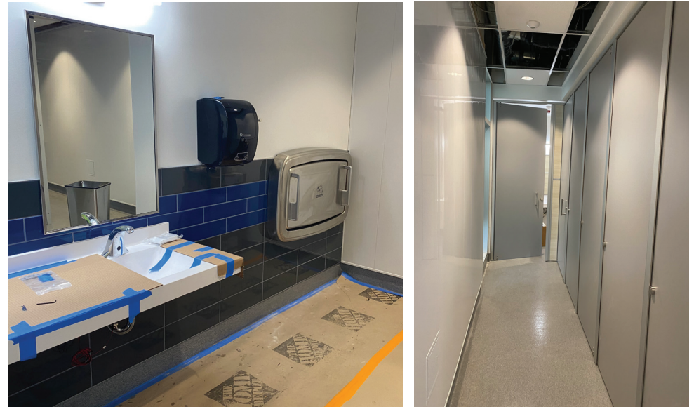
Left: "Trough" sink during construction; Right: New full height toilet partitions
