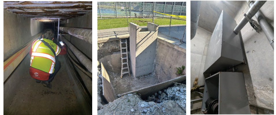
Left: OAI assessing and surveying the utilidor; Middle: New relief opening to provide fresh outside air and improve ventilation within the Utilidor.; Right: Repaired junction box after the source of the incoming water leak was sealed
