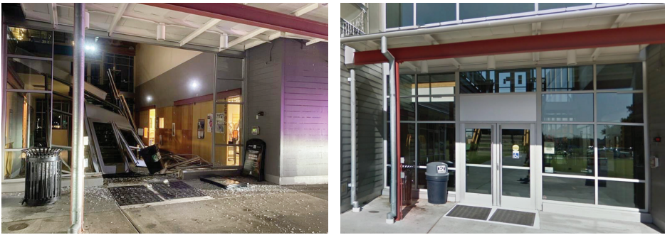
Left: Damaged storefront; Right: Replaced storefront with additional structural support
