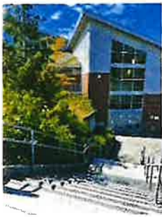
VIEW FROM THE TOP OF THE STAIRS, FACING SOUTHEAST
