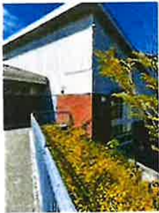
VIEW OF STAIR ENCLOSURE, FACING NORTH
