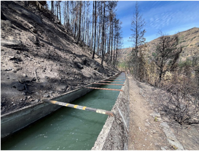
Typical Upper Canal Conditions (Milepost 4.4)
