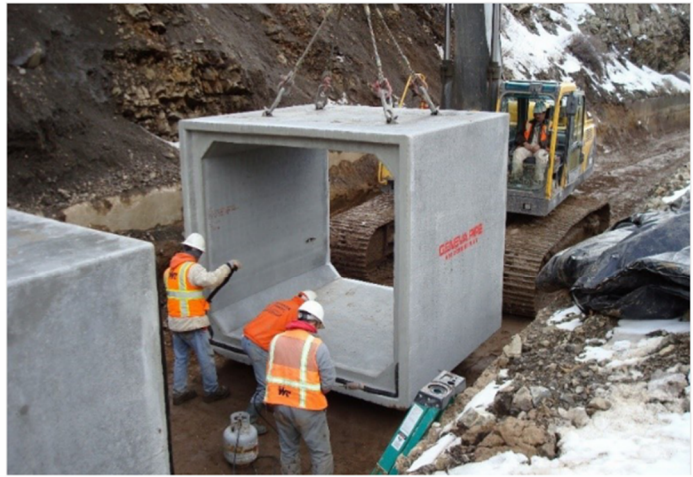
Box Culvert Installation during Winter Months (Courtesy of Whitaker Construction Co.)
