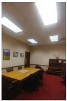
Lower Floor Lighting and a few Conference Spaces – Mostly 2x4 Parabolic Fixtures with T-12 Lamps that were replaced in 1987
