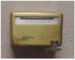
Pneumatic Thermostat (Installed in 1987)
