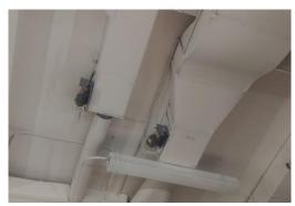
VAV Boxes (box with a pneumatic damper)
