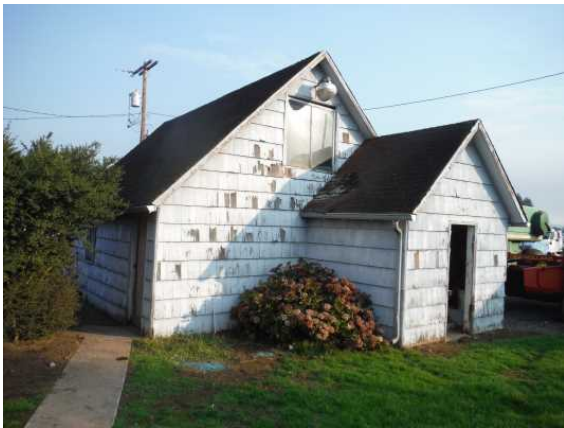
Garage, Viewing Northeast
