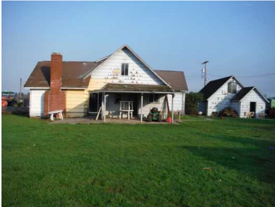
Residence and Garage, Viewing Northeast
