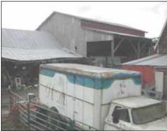
Barn #2 looking west/southwest.
