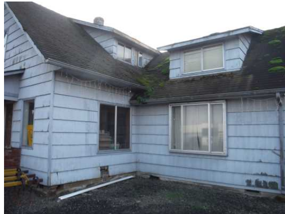
Residence North Facade, Viewing Southeast
