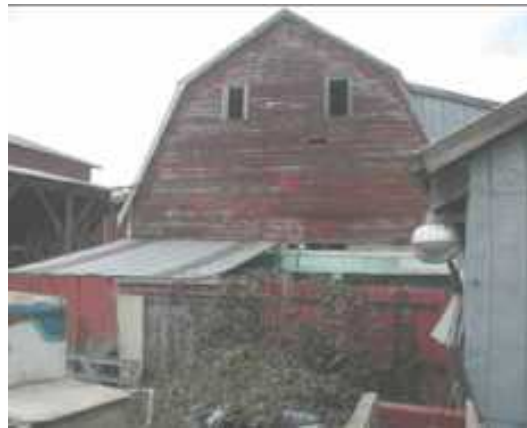
Barn #1 looking west.
