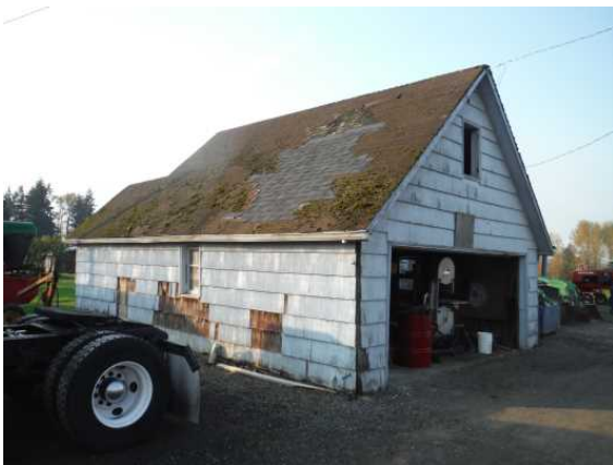
Garage, Viewing Southwest
