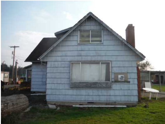
Residence West Elevation, Viewing East
