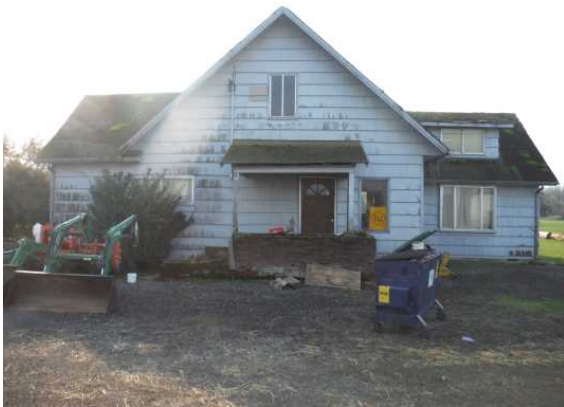
Residence North Facade, Viewing South
