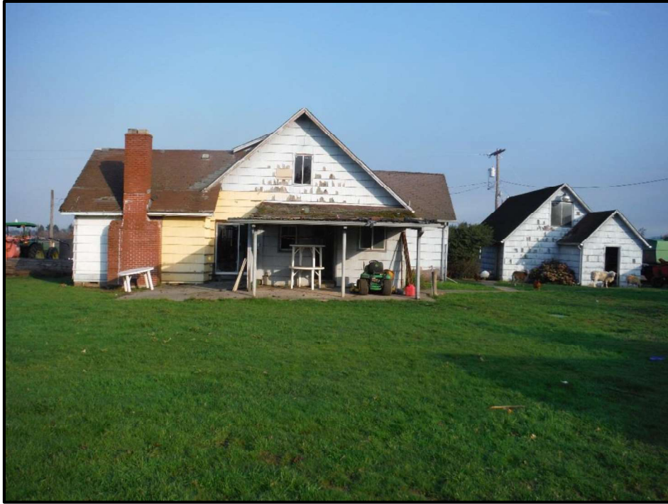
Figure 3. Photograph of the southern elevations of the farmhouse and its detached garage. View is to the north.
