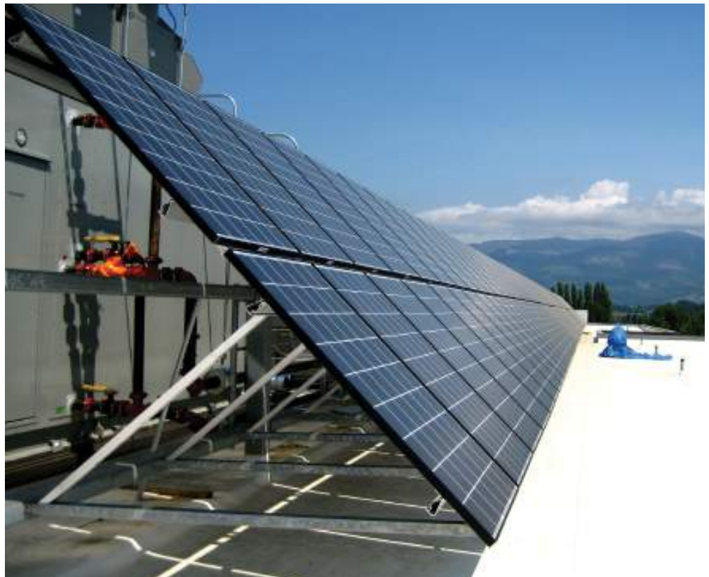
Photovoltaic array, Angst Hall, Skagit Valley College. This system supplies 3% of the building's power.
