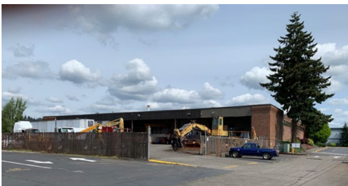
Existing LCC Vocational Building
