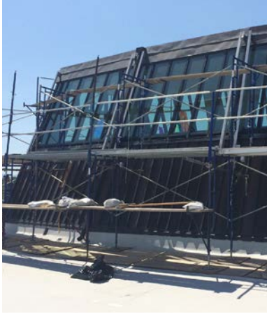
WCC Syre Clerestory - RMC
