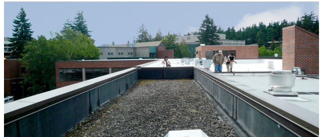
WESTERN WASHINGTON UNIVERSITY | FINE ARTS BUILDING ROOF
