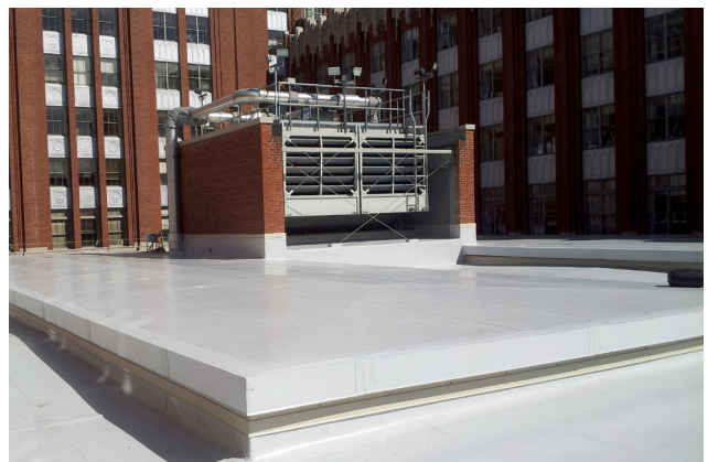
US GSA | FEDERAL OFFICE BUILDING NEW ROOF
