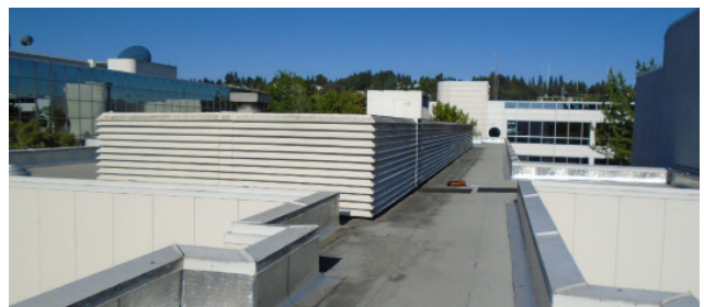
NOAA WRC | ROOF ASSESSMENT
