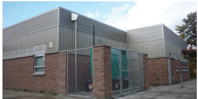
EDMONDS SCHOOL DISTRICT | MEADOWDALE HS GENERATOR
