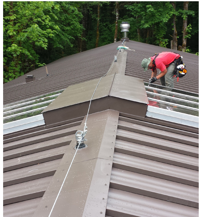
THE EVERGREEN STATE COLLEGE | ROOF ASSESSMENT
