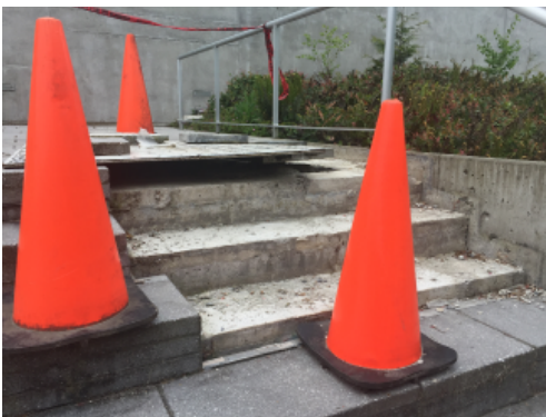
CC Patio stair failure investigation, Cascadia College
