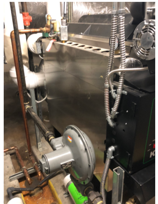
CC2 Boiler Replacement, Cascadia College
