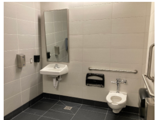
Lynnwood Hall Restroom Remodel & Door Replacement, Edmonds College
