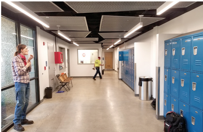
Top: South's renovated Men's locker room Bottom: Welding Building's renovated entry area
