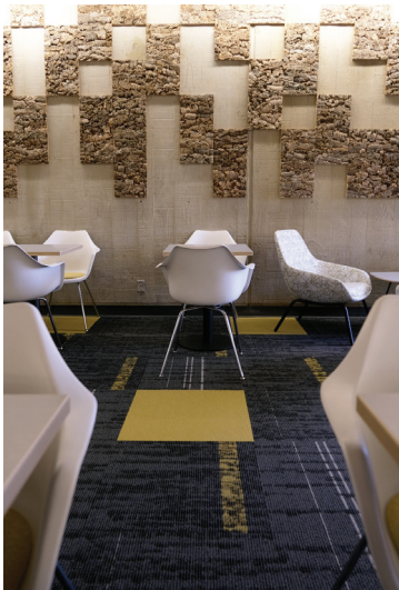
Left: South’s renovated Cafe Alki; Right: Durable cork wall panels used reduce sound within the open space
