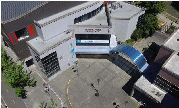
Central’s replaced MAC Canopy
