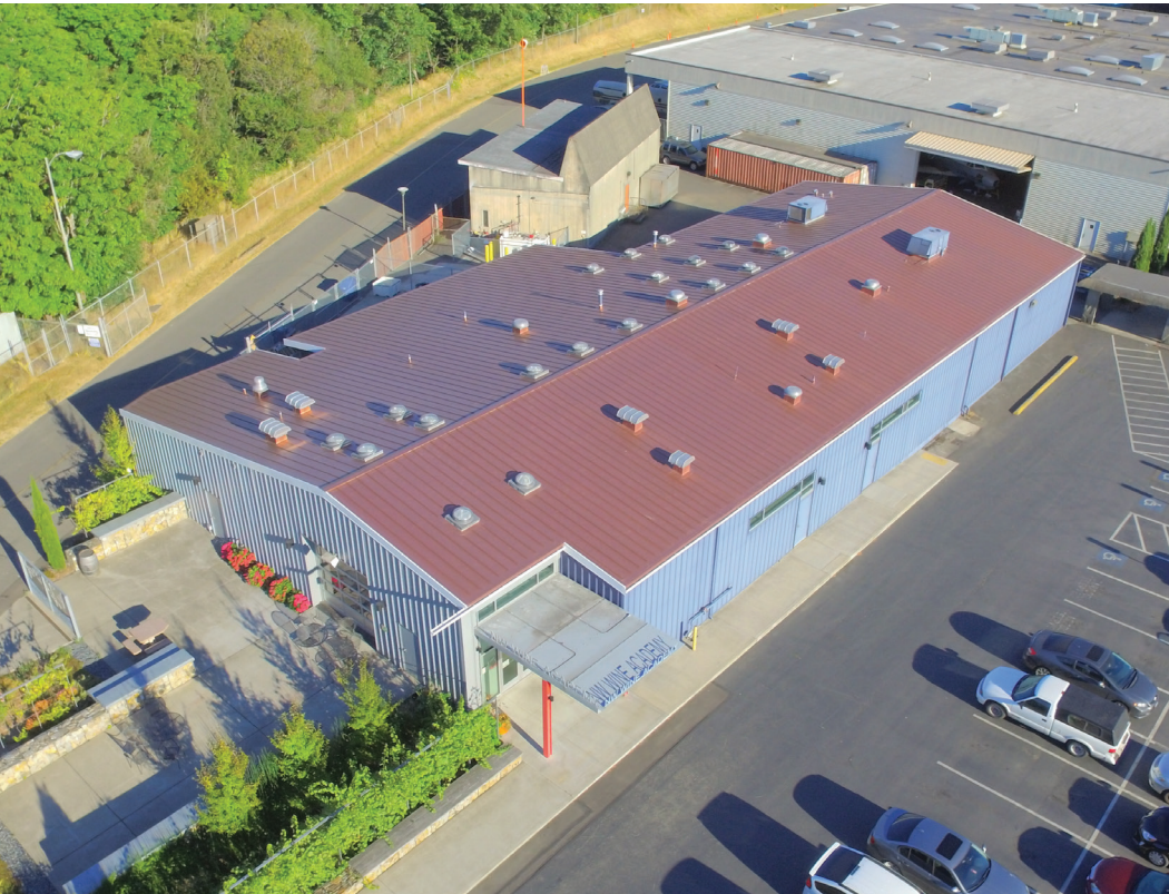
Left: South’s NW Wine Academy’s new PVC over-roof; Top Right: Central’s SVI new roof drain; Middle Right: Central’s Broadway Edison’s lower roof blister repairs; Bottom Right: Broadway Edison’s upper area over-roof
