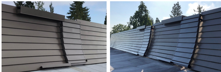
New Mansard Screen Doors at 1800 Bldg. (Left) and 1500 Bldg. (Right)
