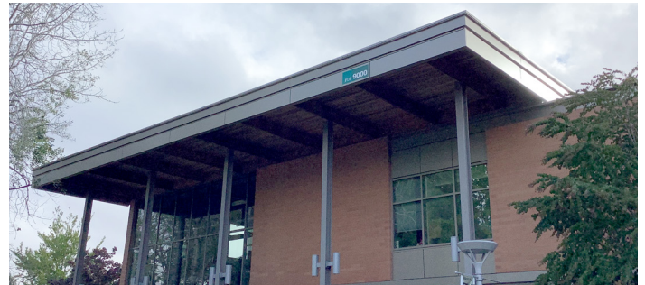
Top: 3000 Bldg. Mansard Replacement; Middle: 1600 Bldg. Mansard Replacement; Bottom: 9000 Bldg. Glu-lam Cladding Repairs
