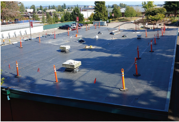
Glacier Hall Roof In-Progress
