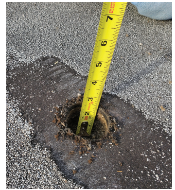
Roof Core Samples Taken
