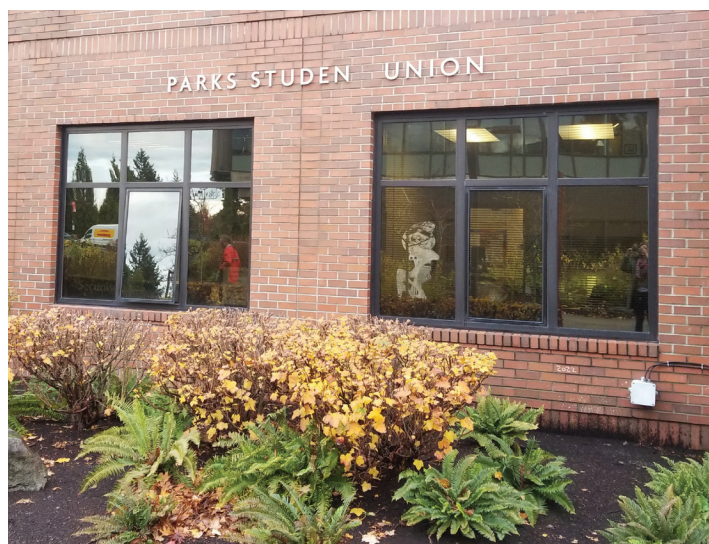
The unit on the left is the test glazing assembly which is now the front entry to the security office suite
