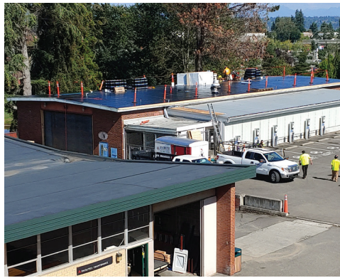
Pilchuck Hall Roof In-Progress
