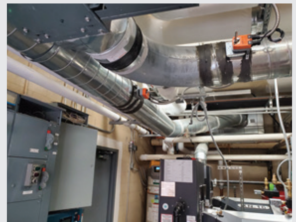
The (2) new 1,600 MBH boilers on see on the right. Existing heating water pumps and boiler flues were retained. New assembly is under warranty to the same manufacturer and to the same installer.
