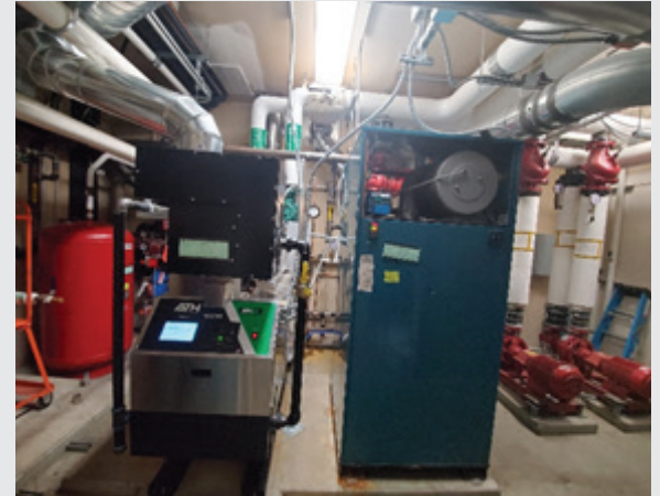
The 1,600 MBH boiler on the left was installed under an Emergency Project. The new boiler was linked to the existing 3,000 on the right so the College would retain heating water redundancy.
