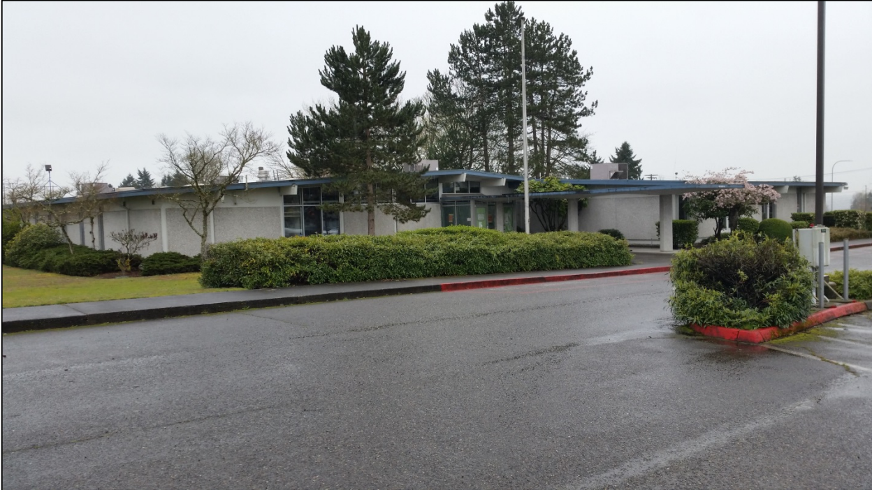
View of the building looking southwesterly.
