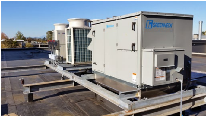
Mechanical Upgrades & Replacements, South Seattle College
