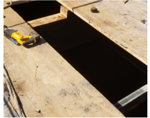
Structural rot repair, Cascade Building Roofing Replacement, Criminal Justice Training Commission
