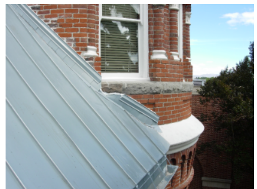
We have completed multiple projects at Central Washington University's iconic Barge Hall. We are currently performing replacement of the building's metal roofing.
