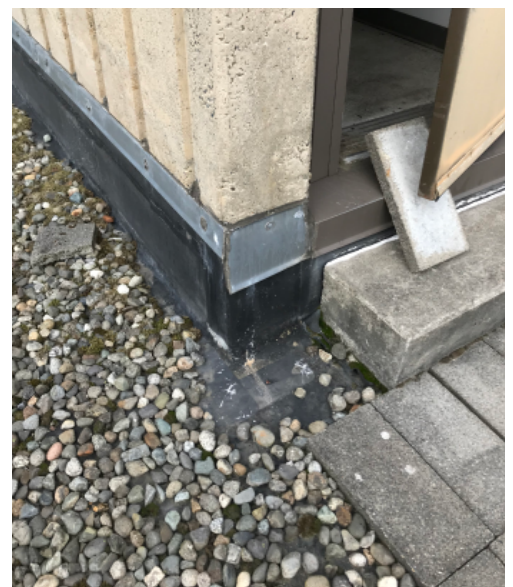
Alderwood Hall roof assessment, Edmonds College
