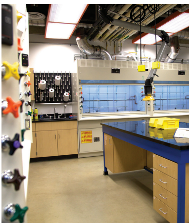
WWU Class & Lab Upgrades - RMC
