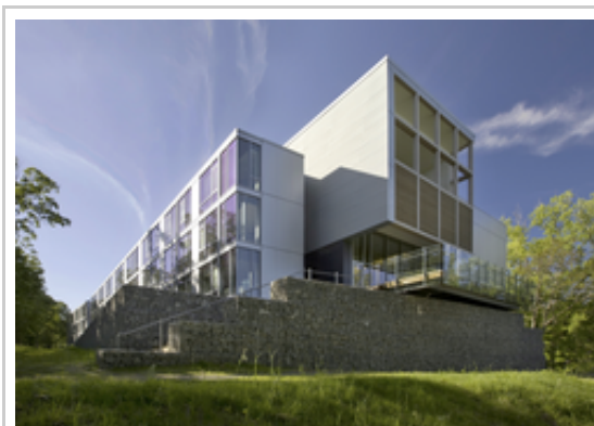
The Gary C. Comer Geochemistry Building at Columbia University features natural ventilation in its office wing; Payette designers took advantage of natural shading from existing trees to keep the building cooler.
