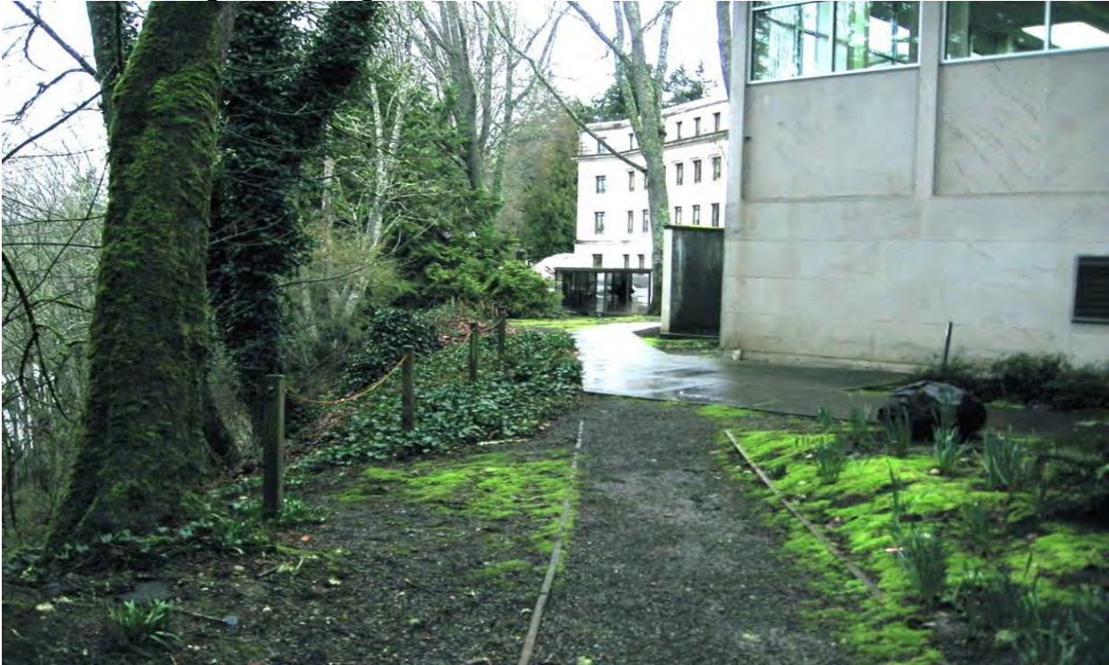
Structural damage to buildings
