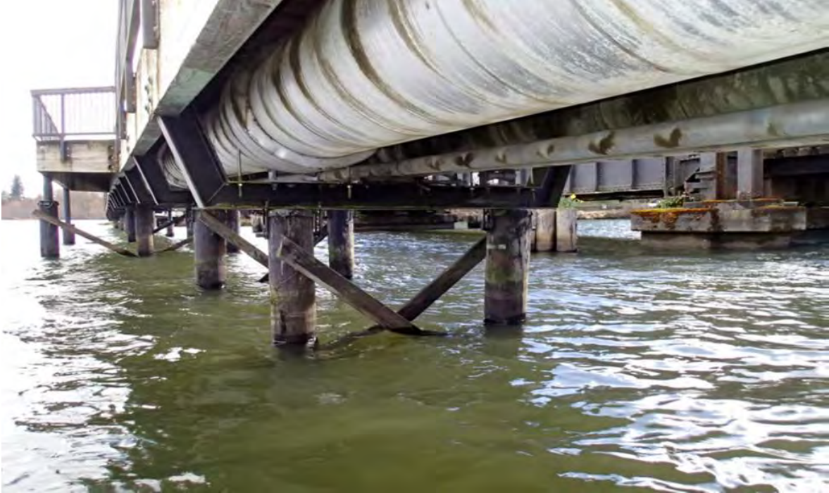
Photo 4 - Typical two-pile pier configuration
