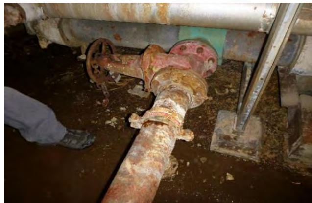
Figure 2: Aged Steam Distribution System
