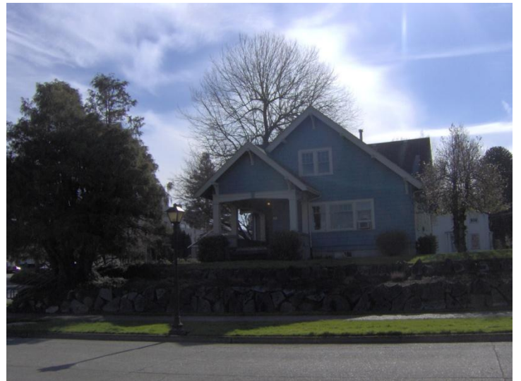
North (Front) Facade
