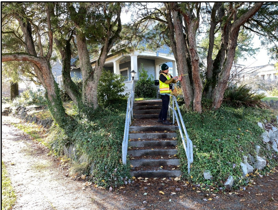
Photo 8. Trees 13-6 (left) and 13-7 (right) growing above rock retaining walls and with concrete steps between.
