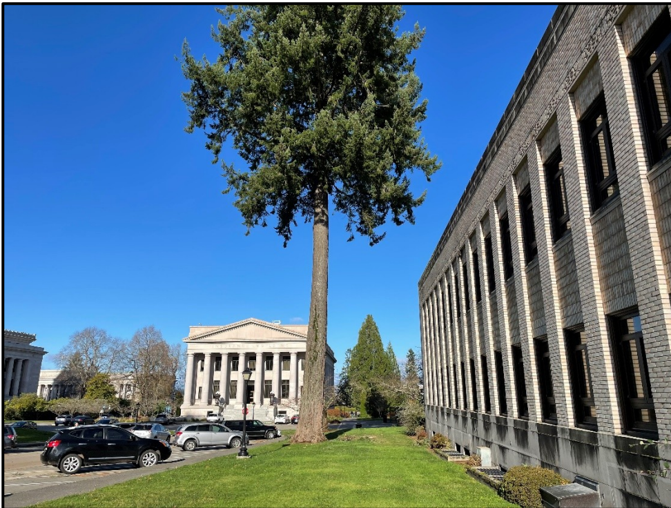
Photo 12. Tree 13-15 in relation to the existing Newhouse Building.
